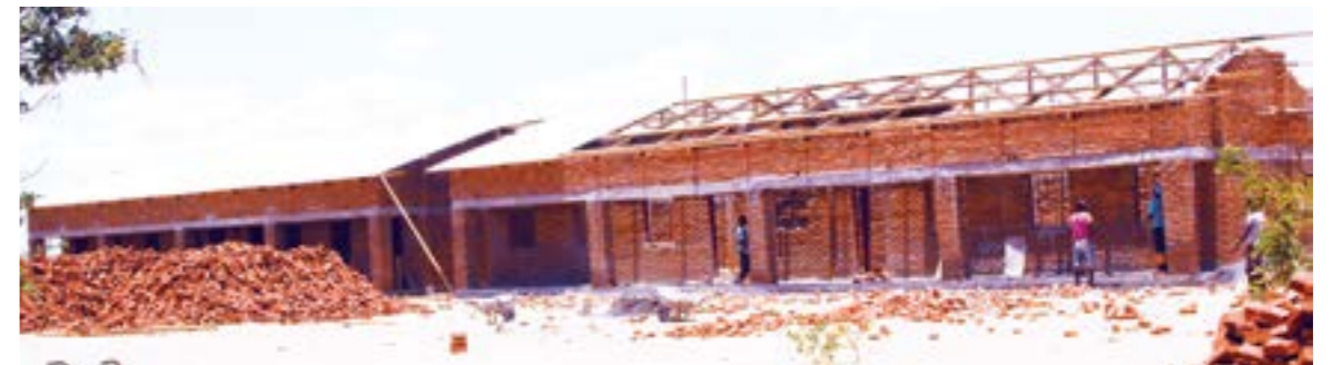
NEW STRUCTURES UNDER CONSTRUCTION.
